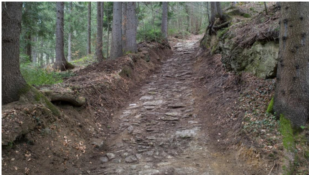
Part of the quarry road paved with marble stones
